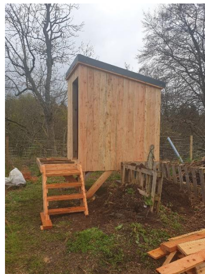
Figure 6: Building the Composting Toilet
